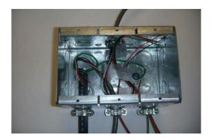
Fig. 3-4 Rough plumbing and wiring to rough-in box, flush mount unit
